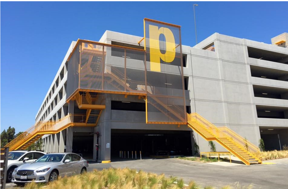
5 Level Parking Structure- Playa Vista, CA
